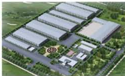
Wujiaqu Industrial Park
